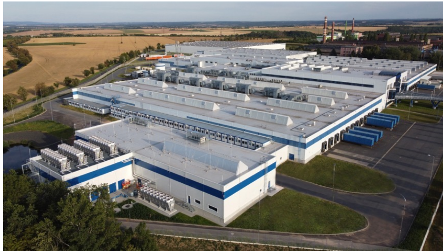
Installation at HPE Grenoble Data Center
